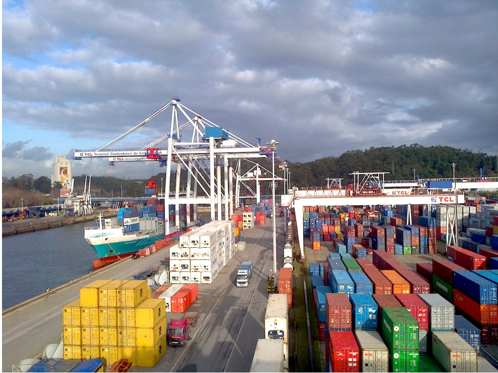
Figure 2.5: Leixões Harbor’s South Terminal as seen from the top of a gantry container crane. Image courtesy of Luís Cabrita [Cab].
