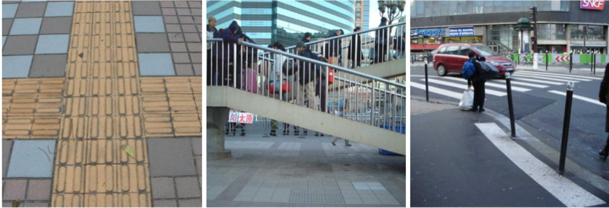
Figure 8.1: (A) Shows two guidance surfaces intersecting without warning in (Taipei, Taiwan) (B) shows a guidance surface leading to stairs without warning in (Beijing, China) (C) shows Incorrect positioning at the entrance to a crosswalk (Paris, France), all example images referenced from [152]
