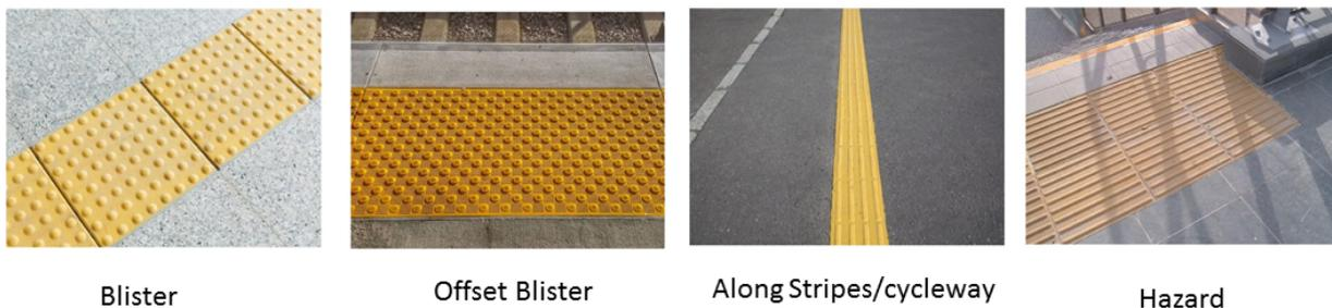
Figure 8.2: Shows most commonly used tactile guidance surfaces for non visual navigation
