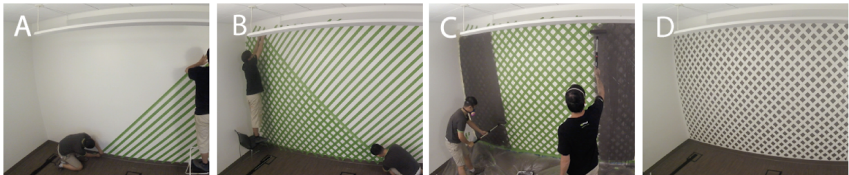
Figure 4.6: Painter’s tape is laid down in a crosshatched pattern (A & B), and then painted en masse with e.g., a roller (C) to create a grid of regular diamonds (D).
